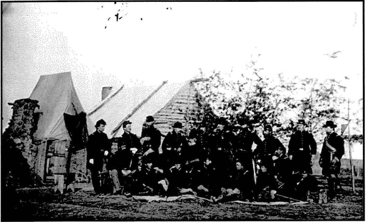
Plate 5. Photograph of the 61 st New York Infantry near Falmouth, depicting the Log Hut Construction.
